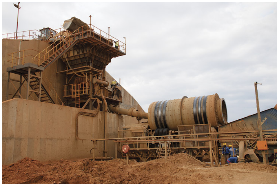
Figure 12. The first step in the wash plant at Fura is the feeding bin (top left), where material enters the washing process. While the material moves down through the bins, water is added and a first screening removes large boulders. The trommel serves a dual function, breaking up clay lumps and screening out oversized materials. This image captures the first of seven steps to reduce the gravel to a concentrate rich in ruby, which is then handled in the sort house. Photo by Wim Vertriest; courtesy of Fura Gems.
