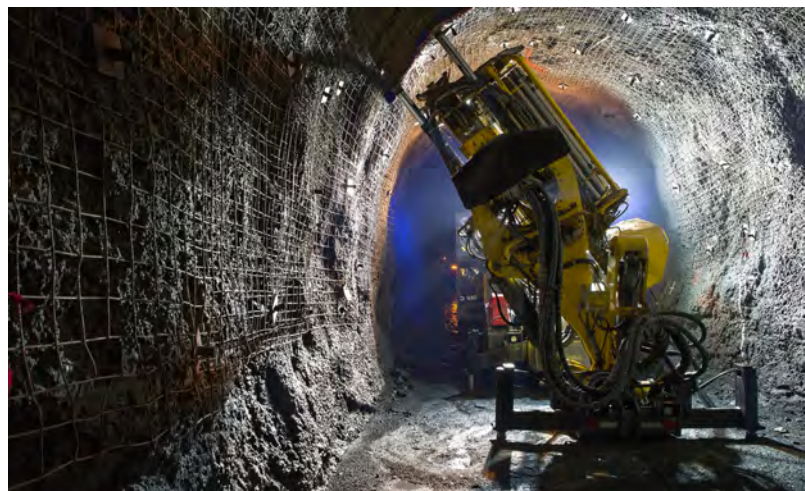
Figure 15. When a tunnel is excavated, this machine is used to install a metal safety screen to prevent debris from falling from the walls or ceiling. Photo courtesy of Diavik Diamond Mine.
