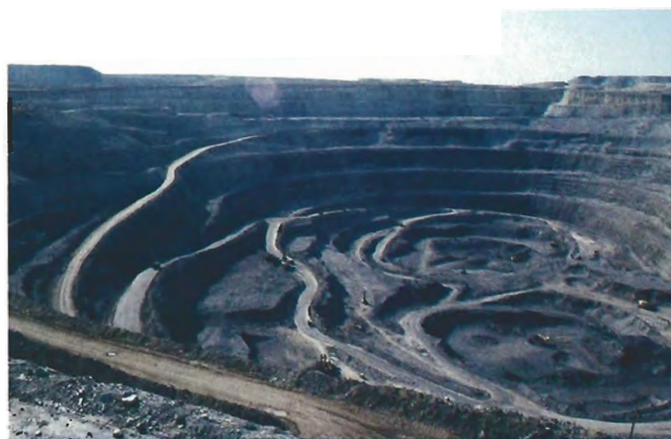
Figure 11. The Udachnaya kimberlite is currently the most important diamond-mining operation in Sakha. It is about 49 acres (20 ha; Johnson et al., 1989) in surface area. Large dump trucks remove the kimberlite and waste rock at a rate of about 1,000 metric tons per hour. The mine operates 24 hours a day and throughout most of the year.
