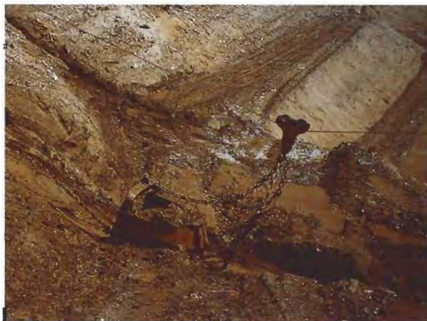
Figure 5. One of two drag scrapers in the larger pit at Capão pulls the saturated, intensely weathered host material to the top for processing. Photo by Daniel A. Sauer.
