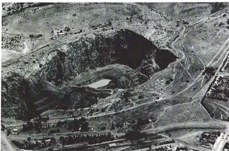
Figure 14. The Premier mine, here shown in an early-20th-century photo, was mined open pit until it closed in 1936. Reopened in 1946 as an underground mining operation, it is still being actively worked. Photo courtesy of De Beers.
