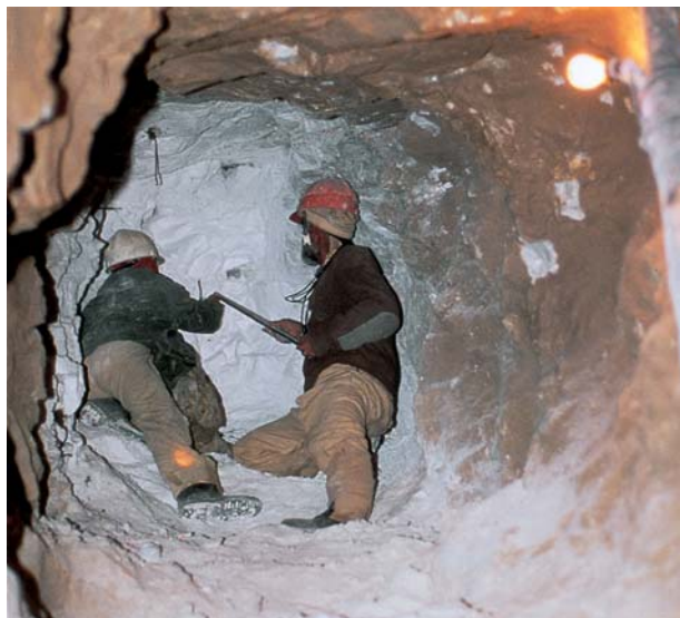
Figure 17. The lower of the two Kashmir ruby deposits has been developed by underground workings with conventional tunneling, using drilling and blasting. Photo by Robert E. Kane.
